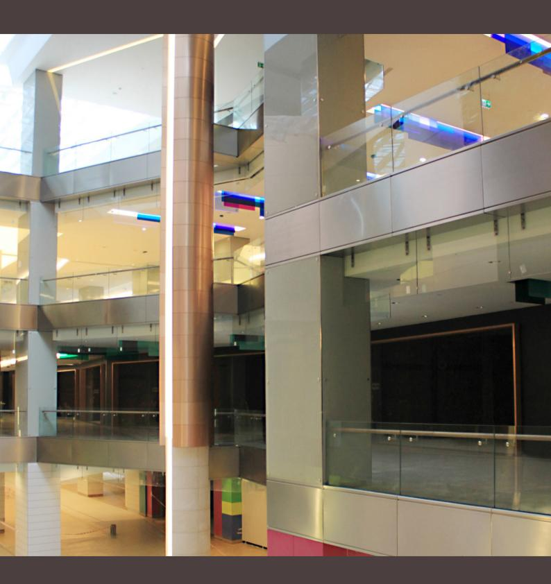
• stainless steel facade cladding integrated with steel construction
